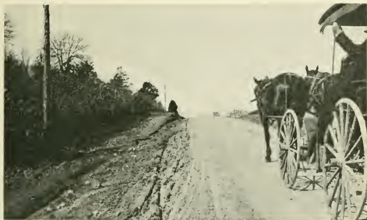
Same road after improvement
